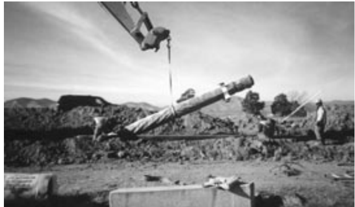
Zone 1 Water Line Replacement Project Construction
